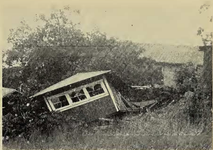
FIG. 4. Overthrown shop building at Kaimalino, from the south.
